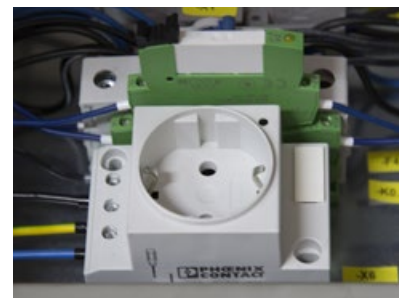
Integrated in the front drawer's control unit, the electrical socket provides easy grid access for servicing equipment.
